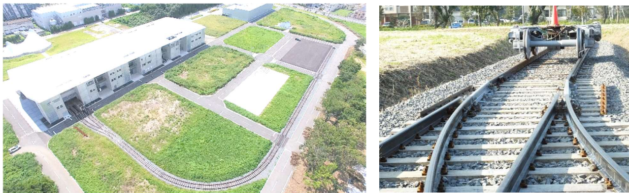
Fig. 3: Over view of Chiba Test Track 2.0 in ITS R&R Experiment Field
